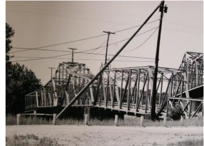
Figure 1.3 Utica Swing Bridge, 1906
